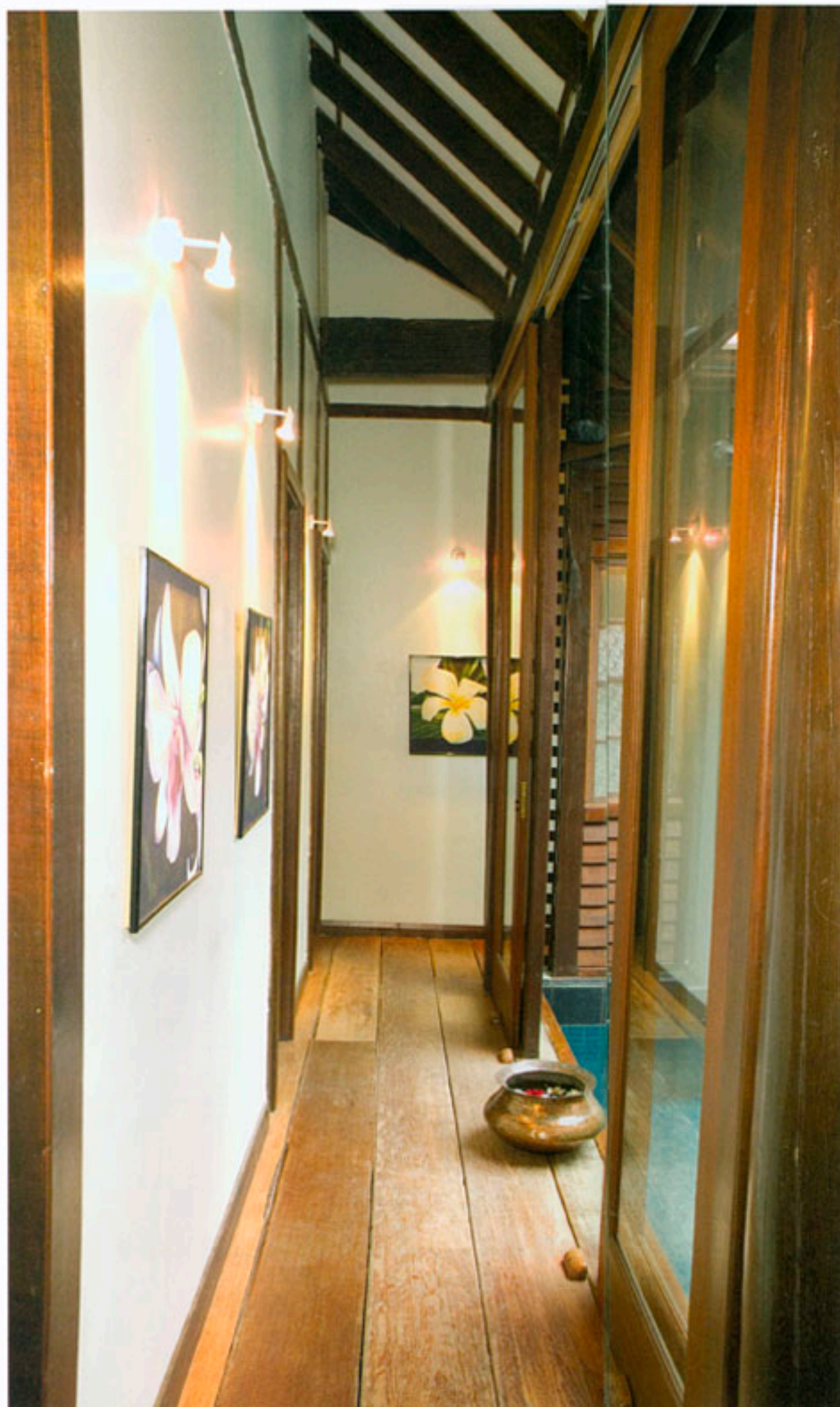
Planks that were 13 inches wide and 5 inches thick with lengths of at least 15 feet were used as flooring in the house.
