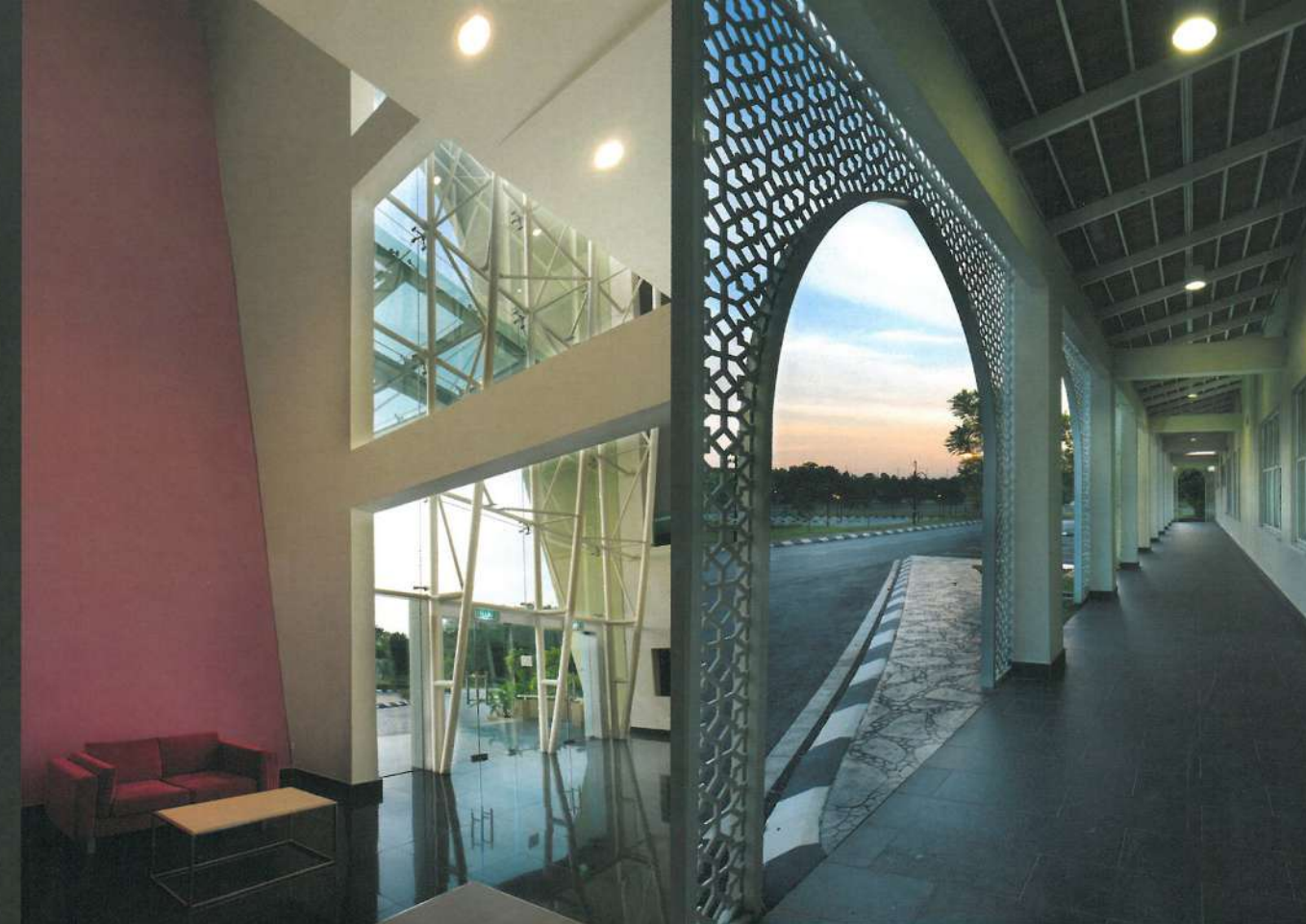
Administration building entrance lobby. The leaning wall in pink, angled lobby and extensive glass wall are supported by the curved steel frame
