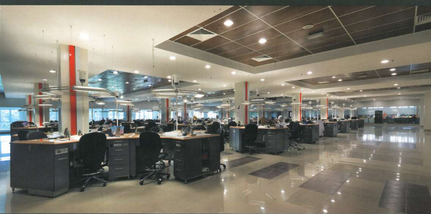
Fabrication lab. The compressed air nozzles in the fabrication lab of 70 proprietary workstations create a lot of noise. Sound insulation was installed in the ceilings to overcome the noise and maintain the clinical cleanliness of the area. No insulating material was installed within the ceiling space that is supported by perforated ceiling boards
